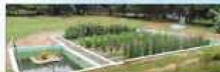
Constructed wetland for waste water treatment
